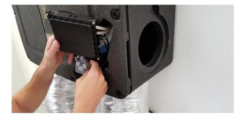
Step 4 • Clean the sensor housing with a dry cloth to clear all the openings.
