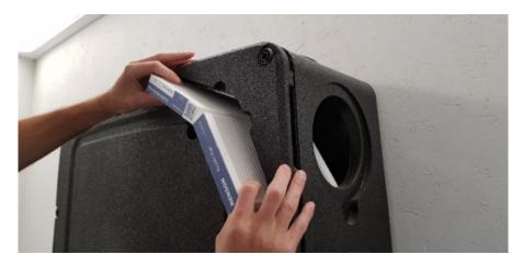
**Step 2** • Clip the connection box out of its socket (if you can remove one of the side caps, you may have easier access to go directly to step 4).
